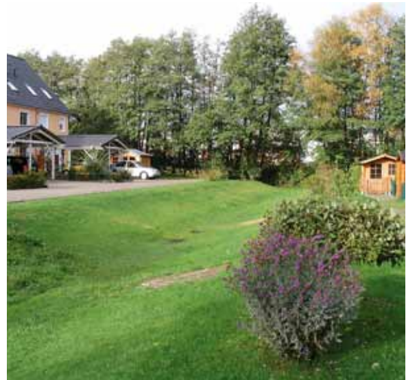
Muldenversickerung in Brokhuchting.
