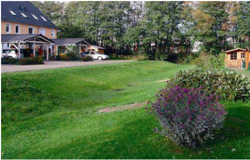
Versickerungsmulde in Brokhuchting
